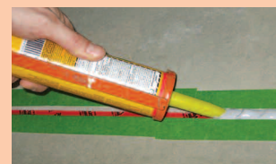
7 Application of flexible adhesive sealant
