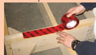
1 Installation on bond-breaking tape
