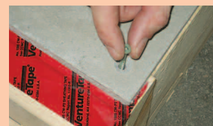
4 Hole must be larger than diameter of screw
